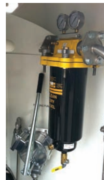
Parker Hannafin filter housing with Facet 0.5 micron filter unit
